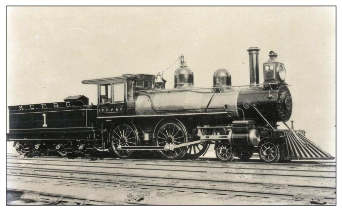
This tall-stacked 4-4-0 No. 1 of Kansas City, Pittsburg & Gulf later became KCS No. 107. It was built in 1895 by Baldwin and scrapped in Shreveport in 1915. The Class B-1 locomotive had 63-inch drivers, 17 inch x 24 inch cylinders, weighed 87,000 pounds with 56,000 pounds on the drivers. Boiler pressure was 160 pounds per sq. inch and tractive effort was 16,377 pounds. The Kansas City, Pittsburg & Gulf relied on 20 of these Baldwin-built locomotives for passenger service and light freight work.
